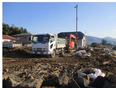
Photo: Mashiki Town removal of the collapsed houses underway .
