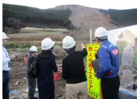
Photo: Collapsed slope
